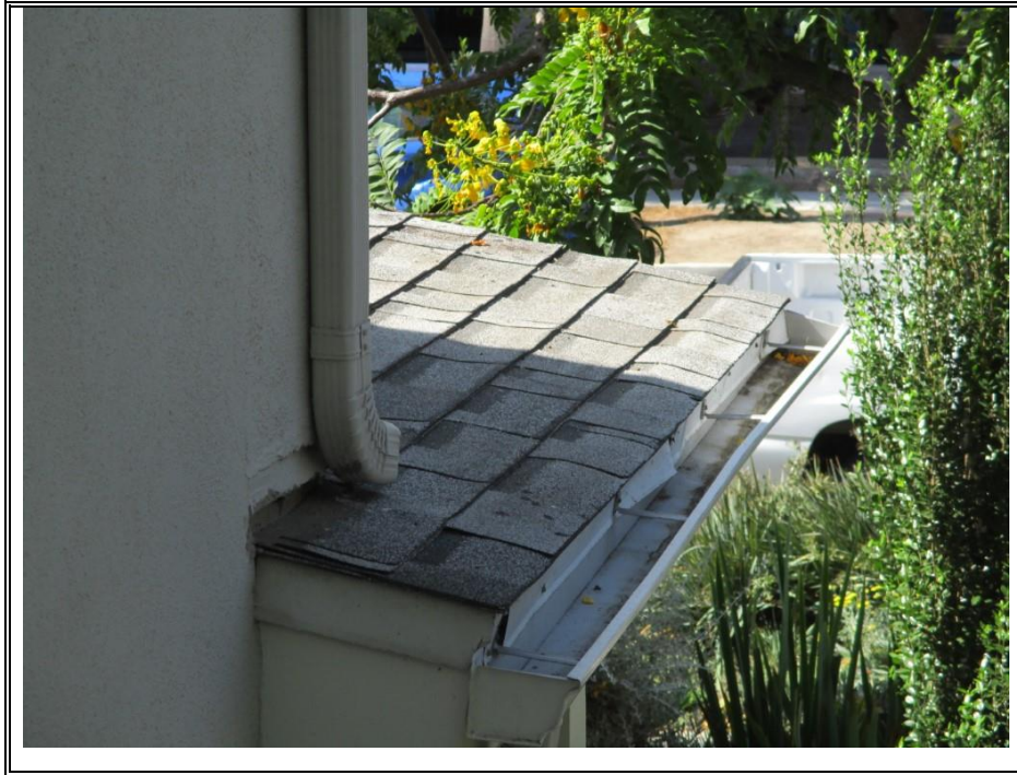
COMPOSITION SHINGLE ROOF (TYPICAL)
