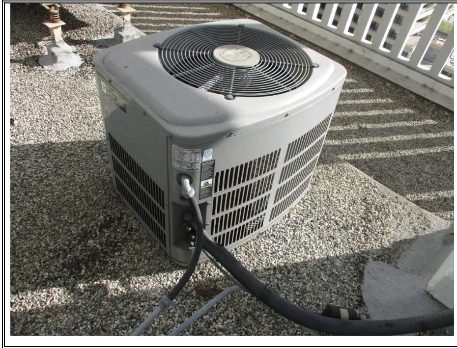
HEAT PUMPS-CONDENSERS (TYPICAL)
