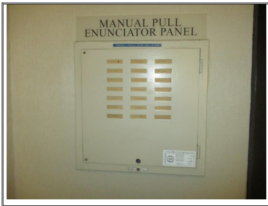
FIRE ANNUNCIATOR SYSTEM (TYPICAL)
