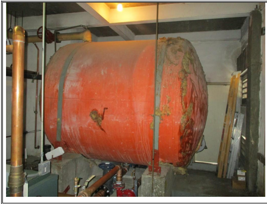
HOT WATER STORAGE TANK (TYPICAL)
