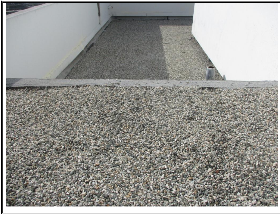
BUILT-UP ROOF (TYPICAL)
