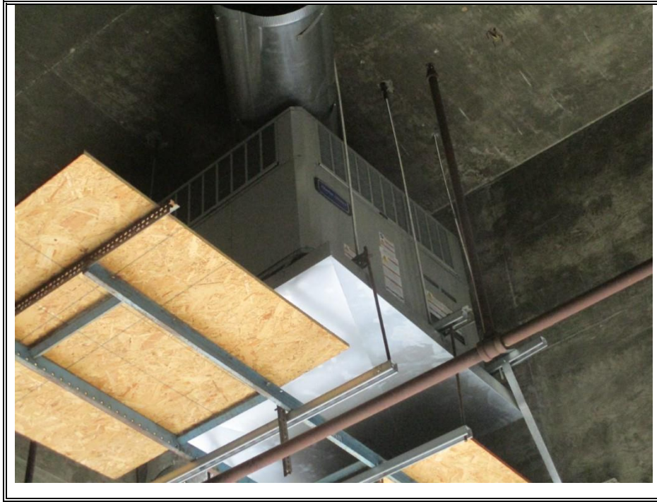
HEAT PUMPS-DUAL PACKS (TYPICAL)
