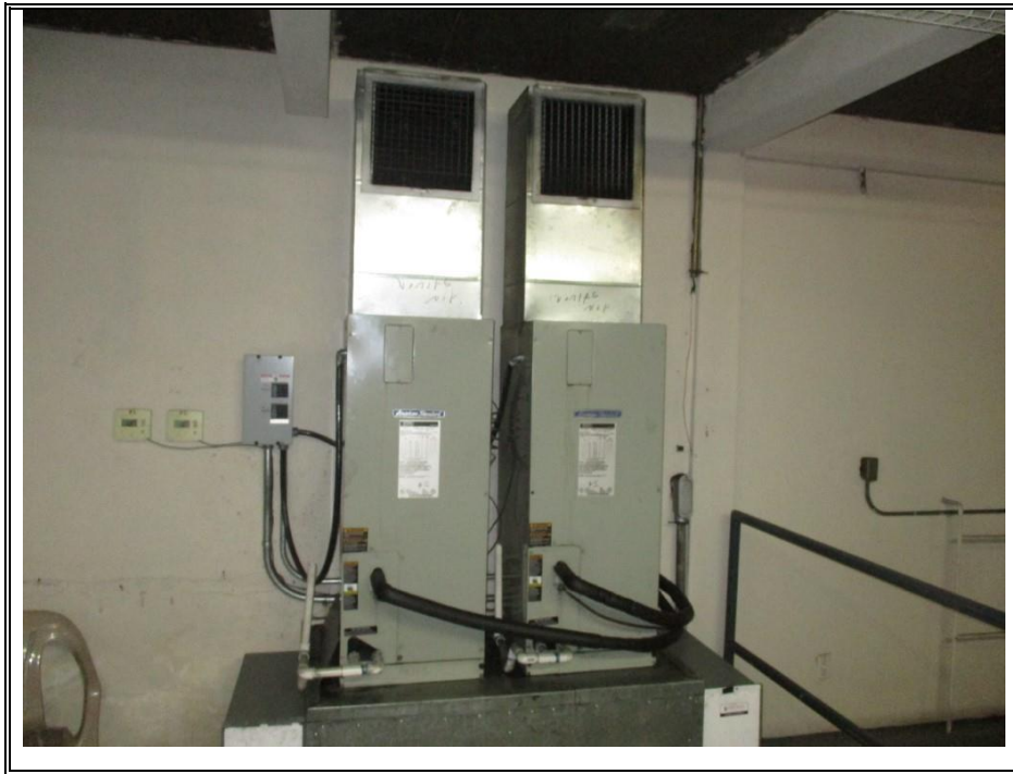
HEAT PUMPS-EVAPORATIVE COILS (TYPICAL)
