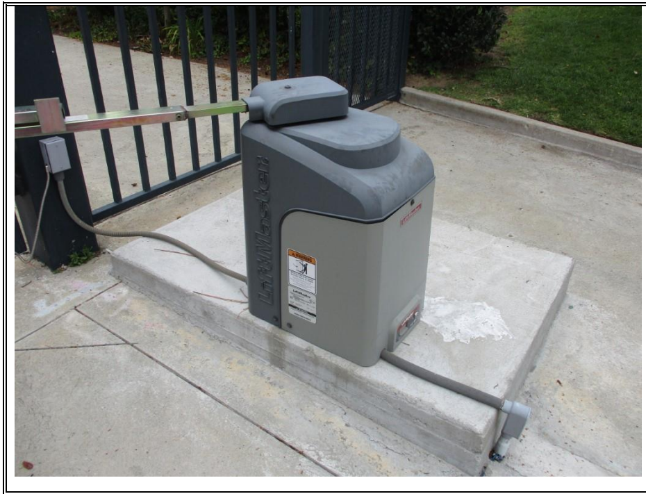
GATE OPERATORS-SWING ARM (TYPICAL)
