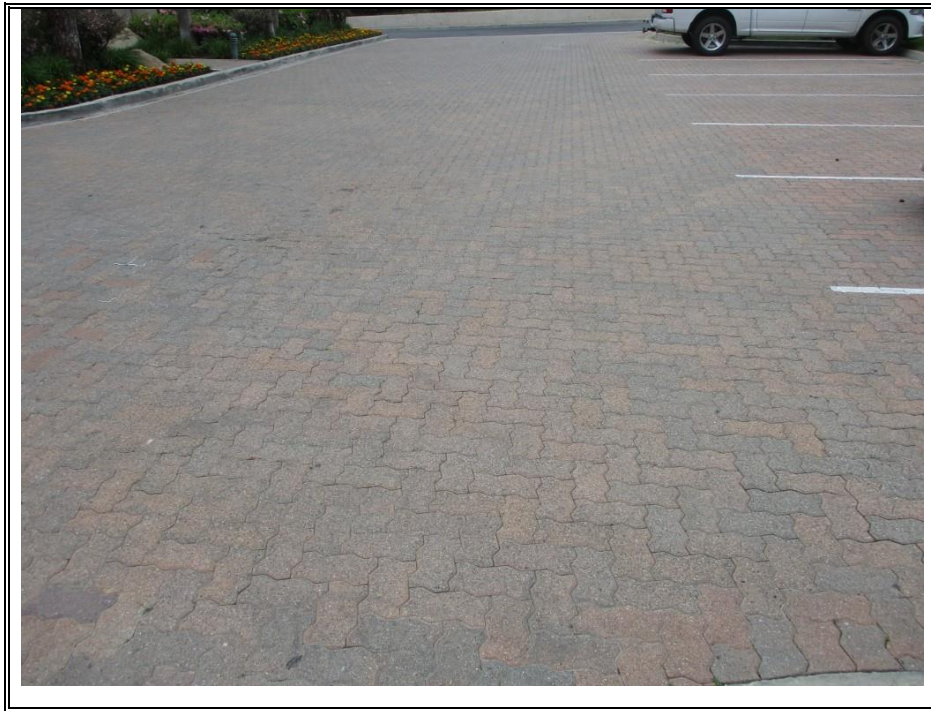
CONCRETE PAVERS – PARKING LOT (TYPICAL)
