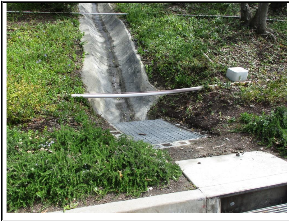
BENCH/DOWNDRAINS (TYPICAL)
