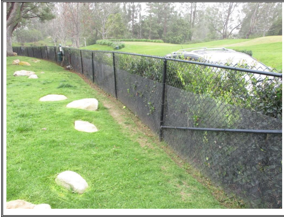
CHAIN LINK FENCING (TYPICAL)
