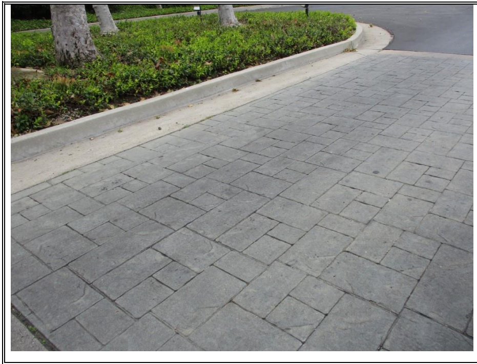
STAMPED CONCRETE (TYPICAL)
