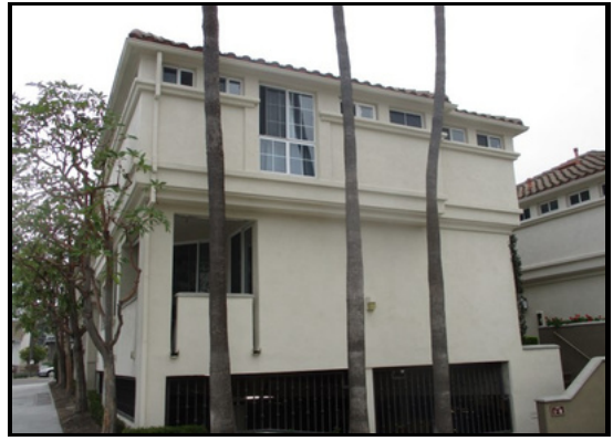
Center deck does not protrude, therefore, likely exempted, however, decks to the left do protrude; elevated inspection requirements likely apply.
