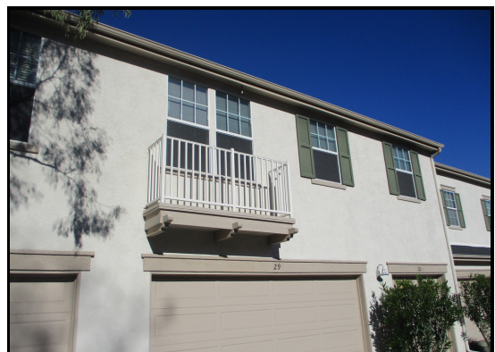
Attached decorative element, not designed for human occupancy; elevated inspection requirements likely does not apply.
