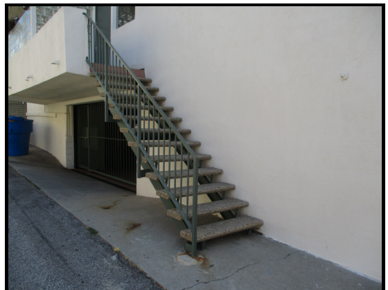
Metal framed stairs likely exempted; however, deck and door landing are wood framed, elevated inspection requirements likely apply.
