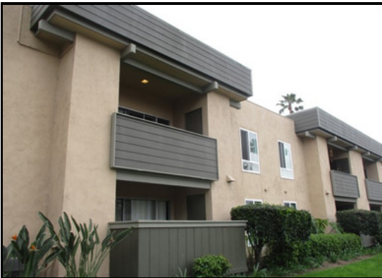
Elevated deck does not protrude; elevated inspection requirements likely does not apply.
