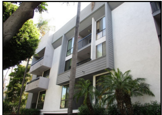
Elevated deck does not protrude; elevated inspection requirements likely does not apply.
