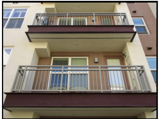
Wood framed, elevated, railings subject to fallibility. Note the presence of ventilation; inspection requirements likely apply.
