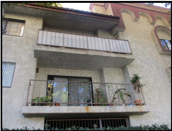
Wood framed, elevated, railings subject to fallibility. Note the lack of ventilation – destined to fail; inspection requirements likely apply.
