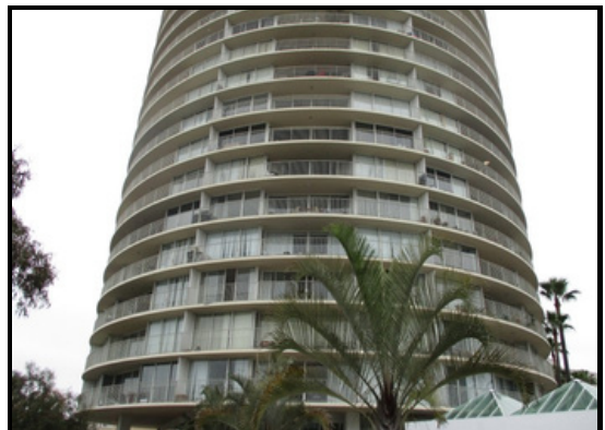
Concrete and steel construction; elevated inspection requirements likely does not apply.
