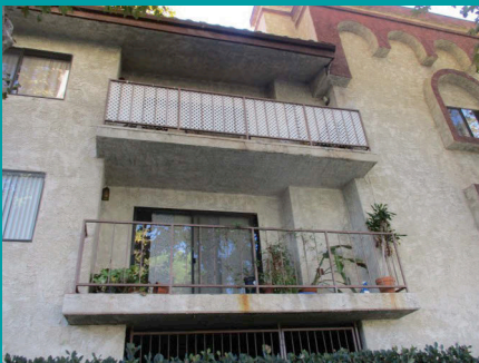
Wood framed, elevated, railings subject to fallibility. Note the lack of ventilation - destined to fail; inspection requirements likely apply.
