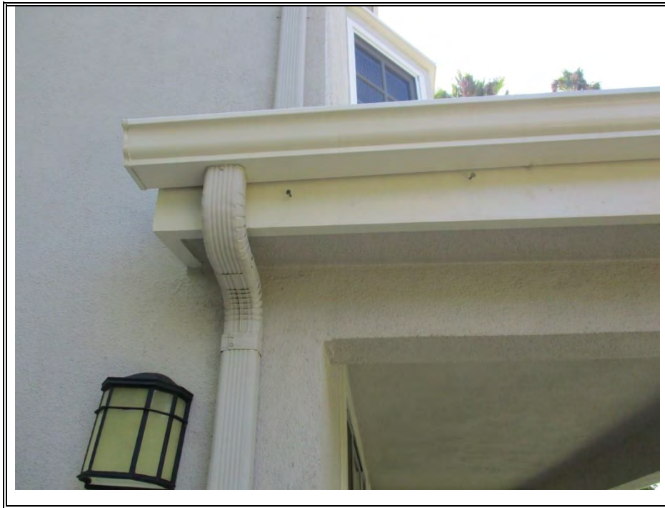
GUTTERS & DOWNSPOUTS (TYPICAL)
