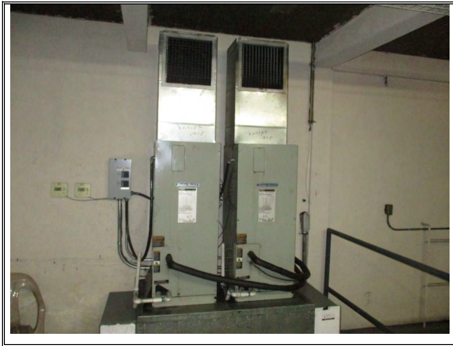
HEAT PUMPS-EVAPORATIVE COILS (TYPICAL)
