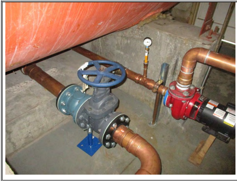
CIRCULATION PUMPS (TYPICAL)
