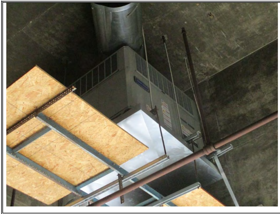
HEAT PUMPS-DUAL PACKS (TYPICAL)
