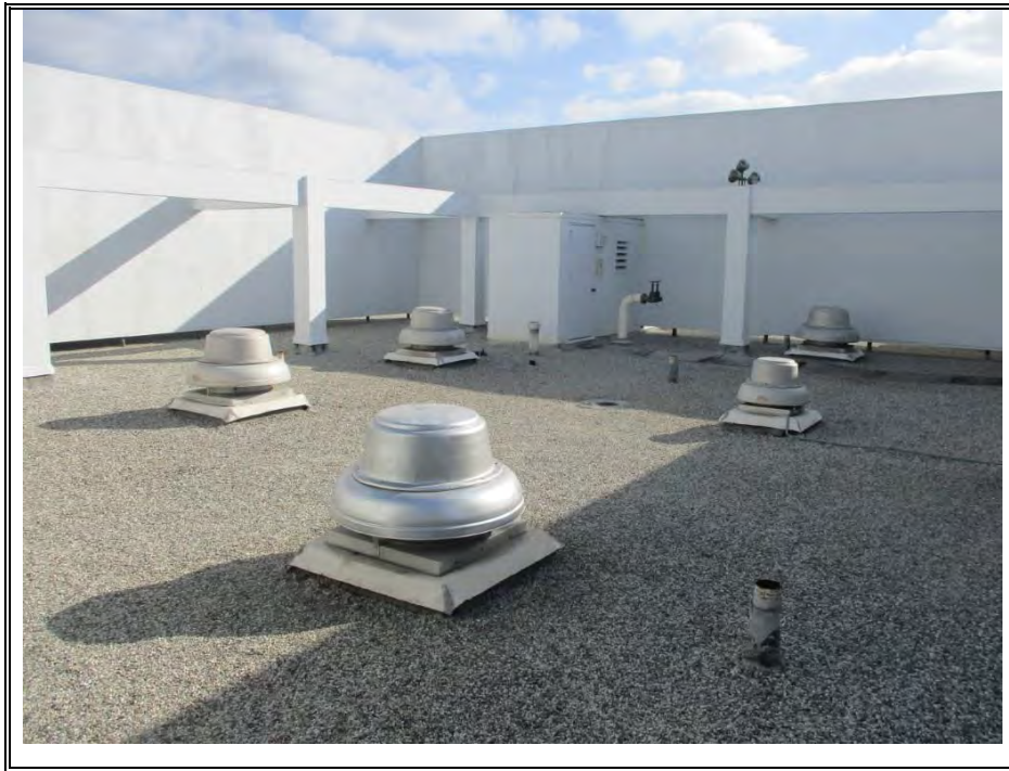
EXHAUST FANS-INTERIORS (TYPICAL)
