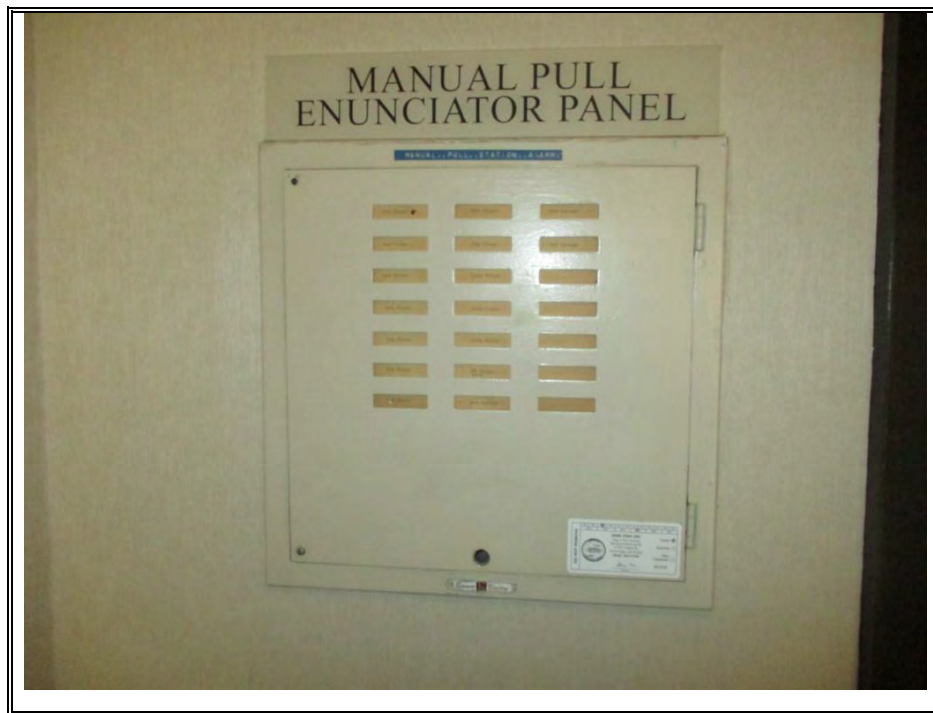
FIRE ANNUNCIATOR SYSTEM (TYPICAL)
