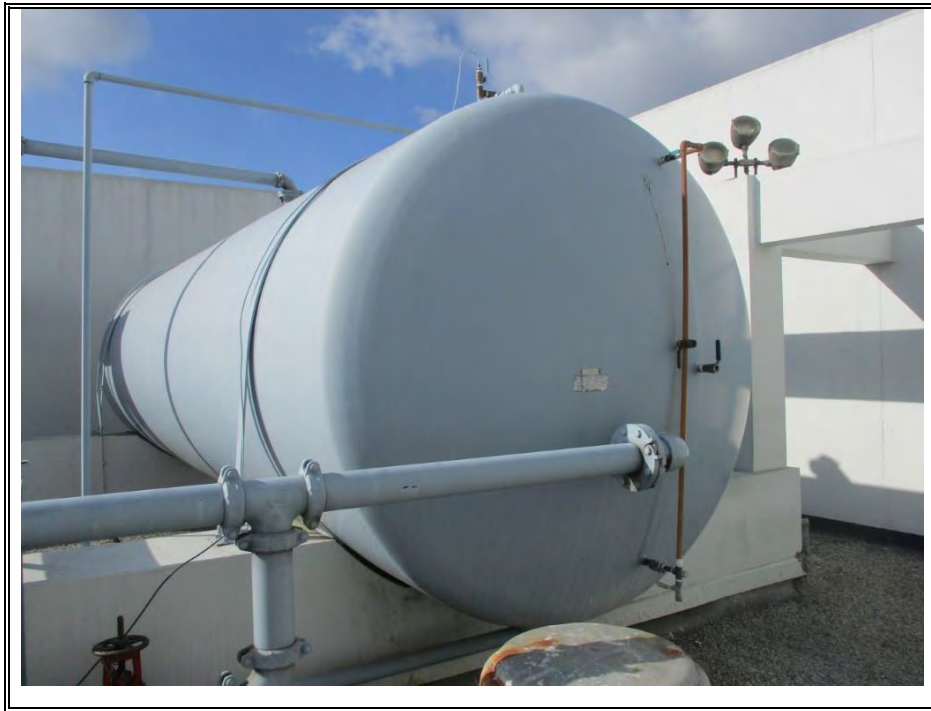
COLD WATER STORAGE TANK-RELINING (TYPICAL)
