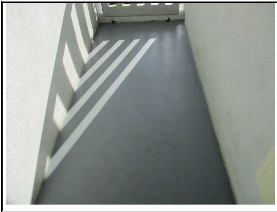
MEMBRANE DECKS-COMMON (COATING) (TYPICAL)
