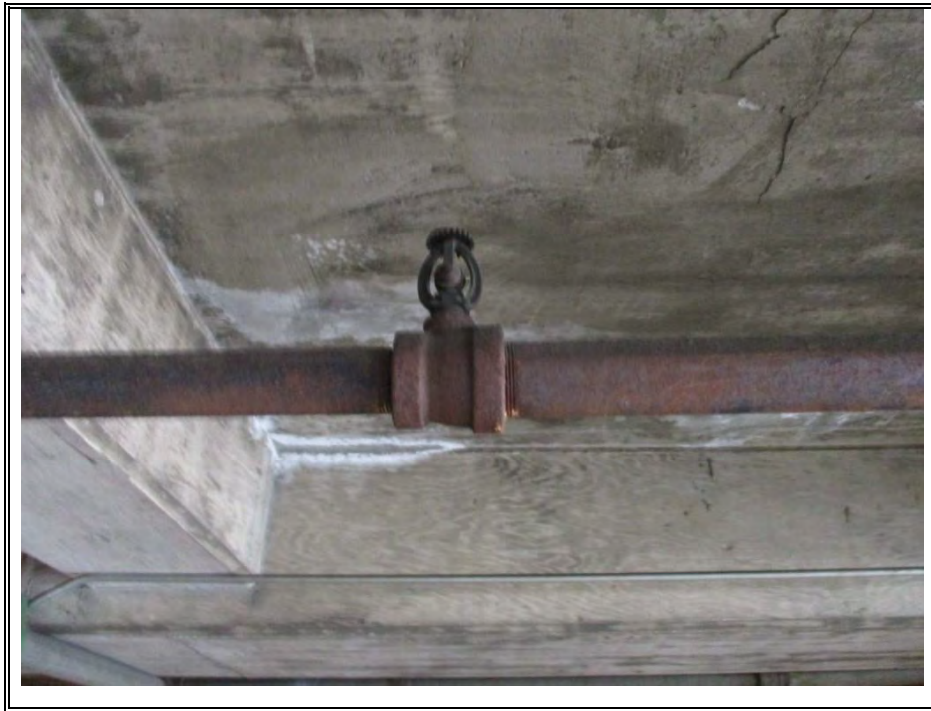
FIRE SPRINKLERS (TYPICAL)
