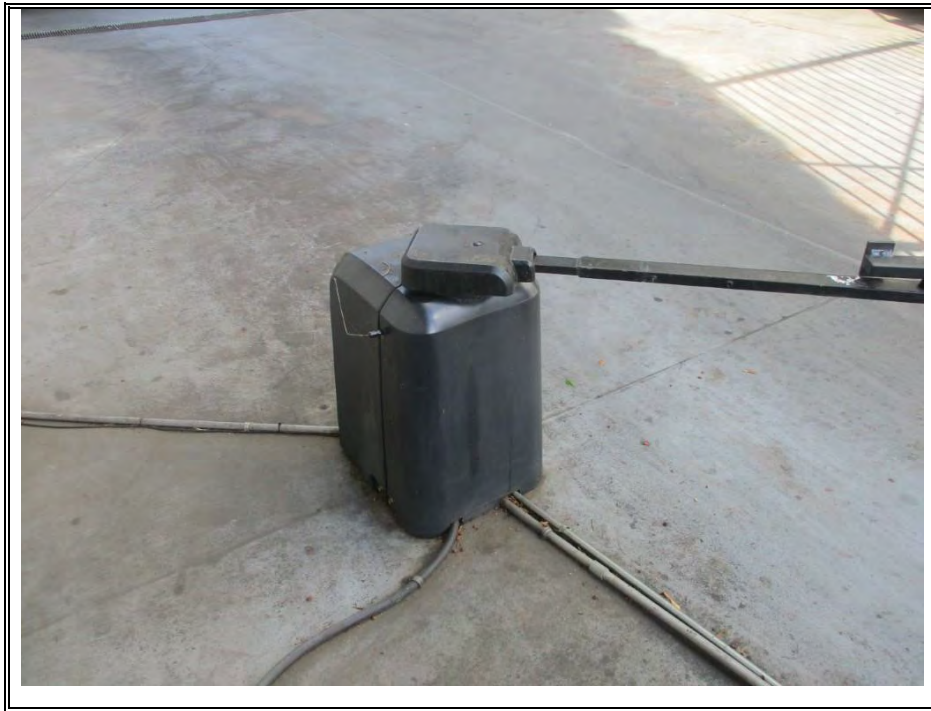
GATE OPERATOR (TYPICAL)
