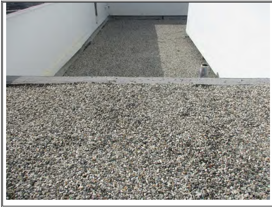
BUILT-UP ROOF (TYPICAL)
