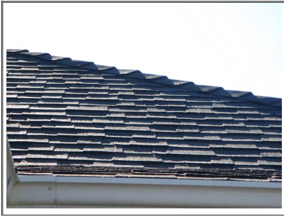
COMPOSITION SHINGLE ROOF (TYPICAL)
