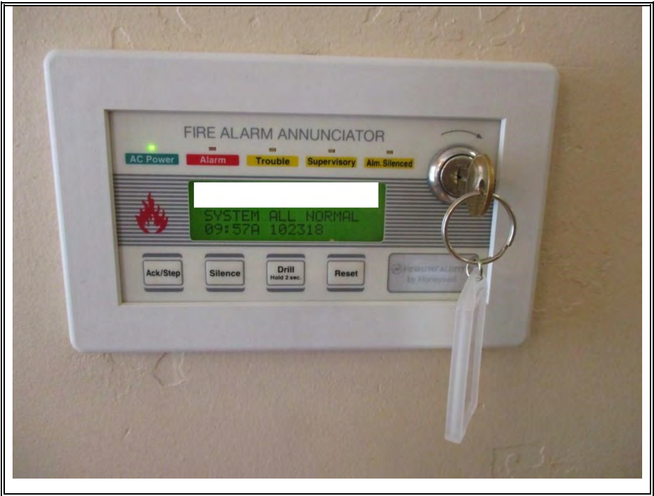
FIRE ANNUNCIATOR SYSTEM (TYPICAL)
