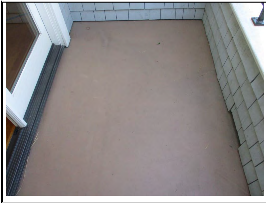
MEMBRANE DECKS-COMMON (COATING) (TYPICAL)
