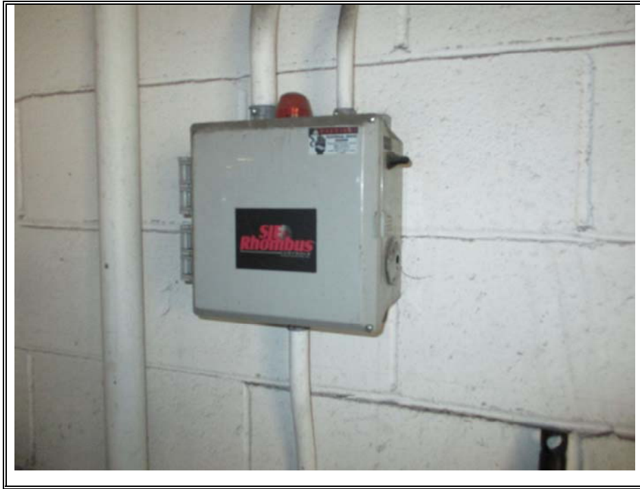
SUMP PUMP CONTROL PANEL (TYPICAL)
