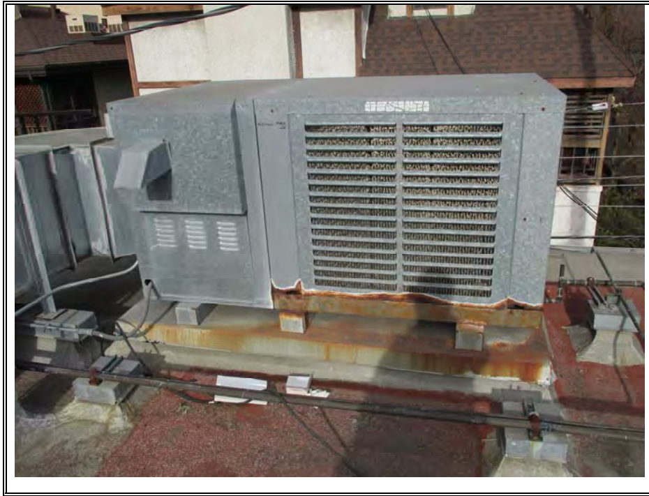
MAKE-UP AIR FAN (TYPICAL)
