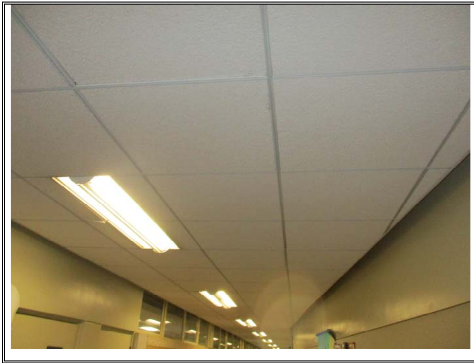
T-BAR CEILING PANELS (TYPICAL)
