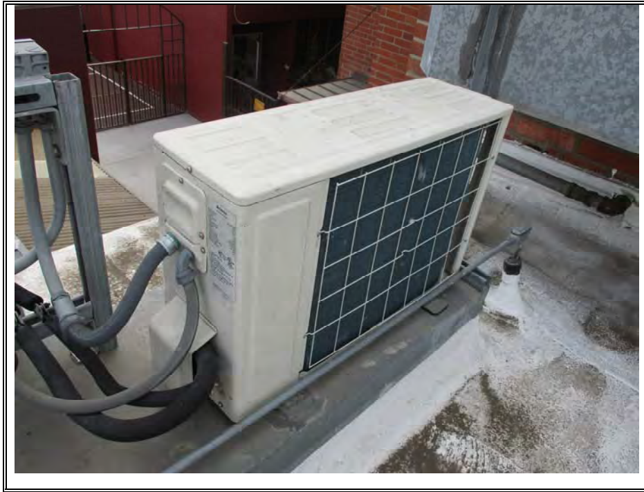
AIR CONDITIONING-CONDENSER (TYPICAL)
