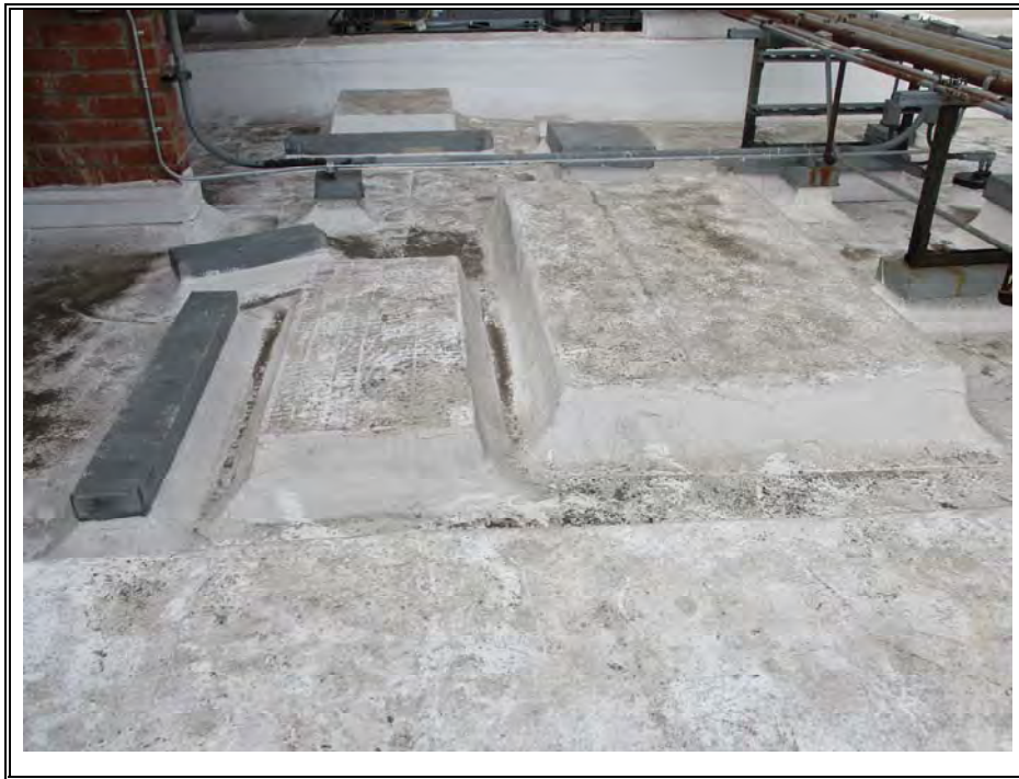
MODIFIED CAP SHEET ROOF (TYPICAL)
