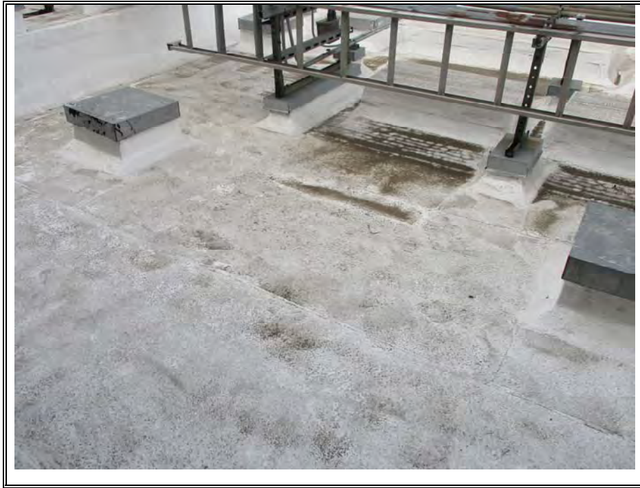
MODIFIED CAP SHEET ROOF-COATING (TYPICAL)
