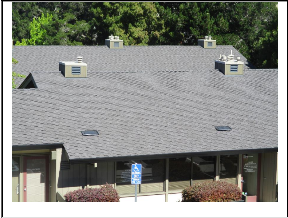
COMPOSITION SHINGLE ROOF (TYPICAL)
