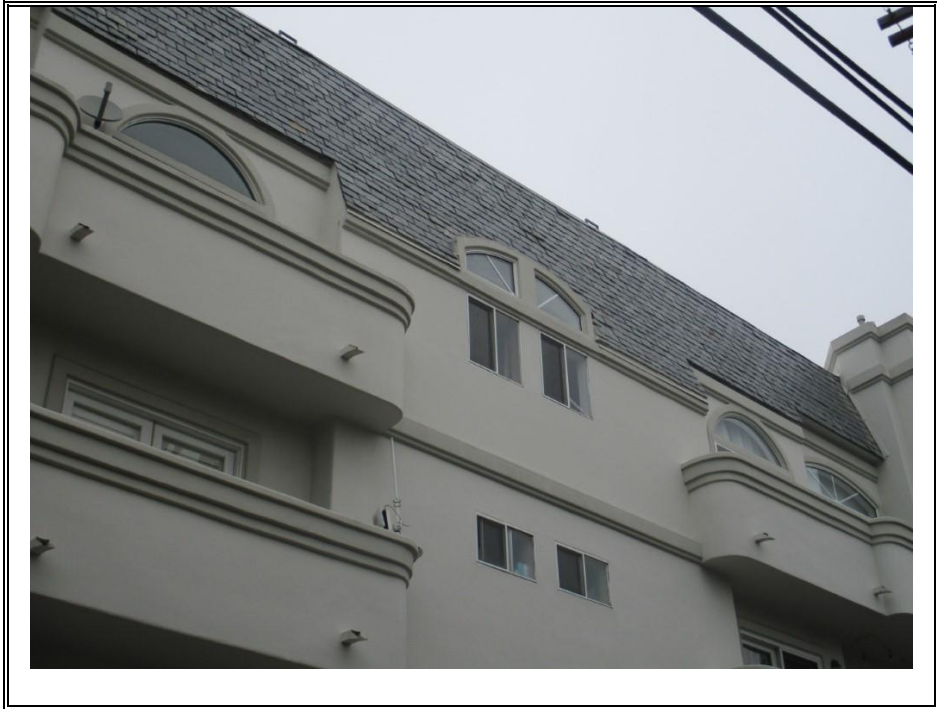
CONCRETE TILE ROOF (TYPICAL)
