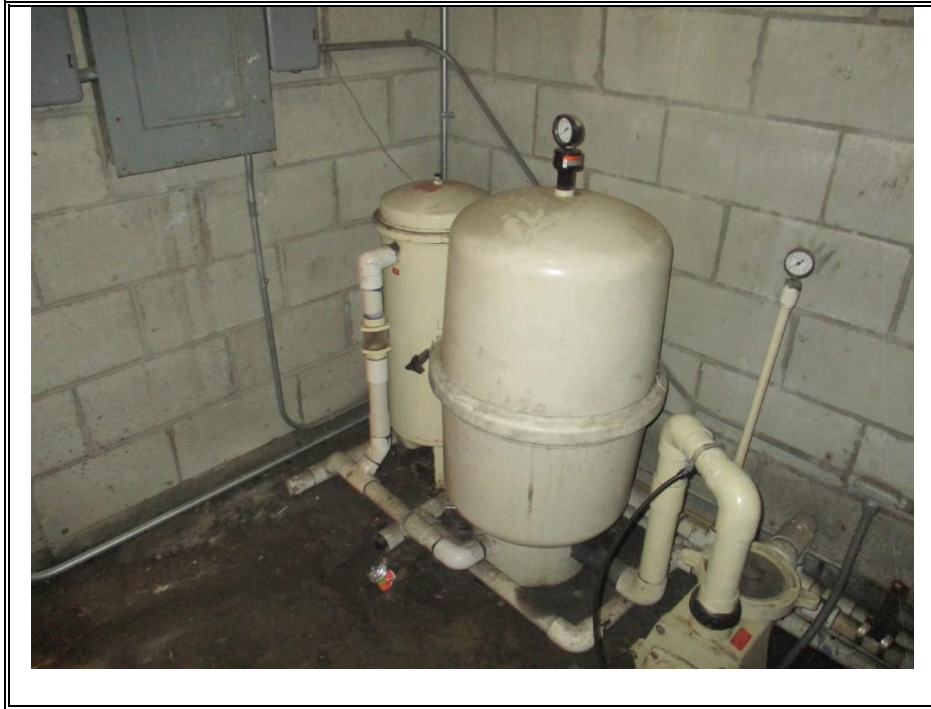
FILTER & SEPARATION TANK (TYPICAL)
