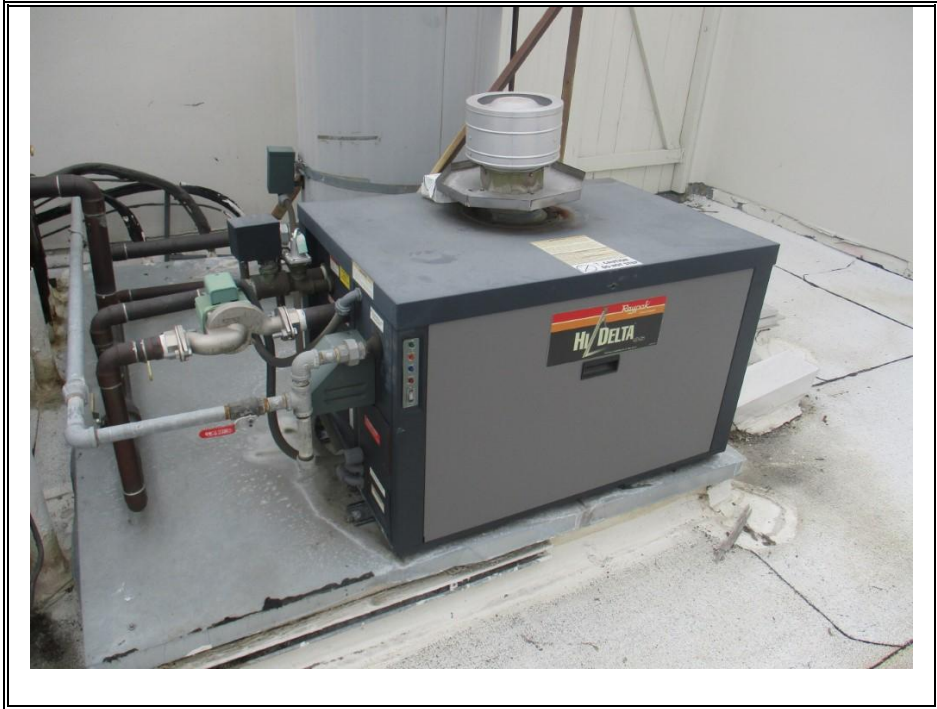
BOILER-REPLACE (TYPICAL)
