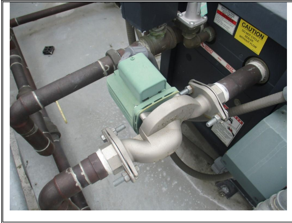
CIRCULATION PUMP (TYPICAL)
