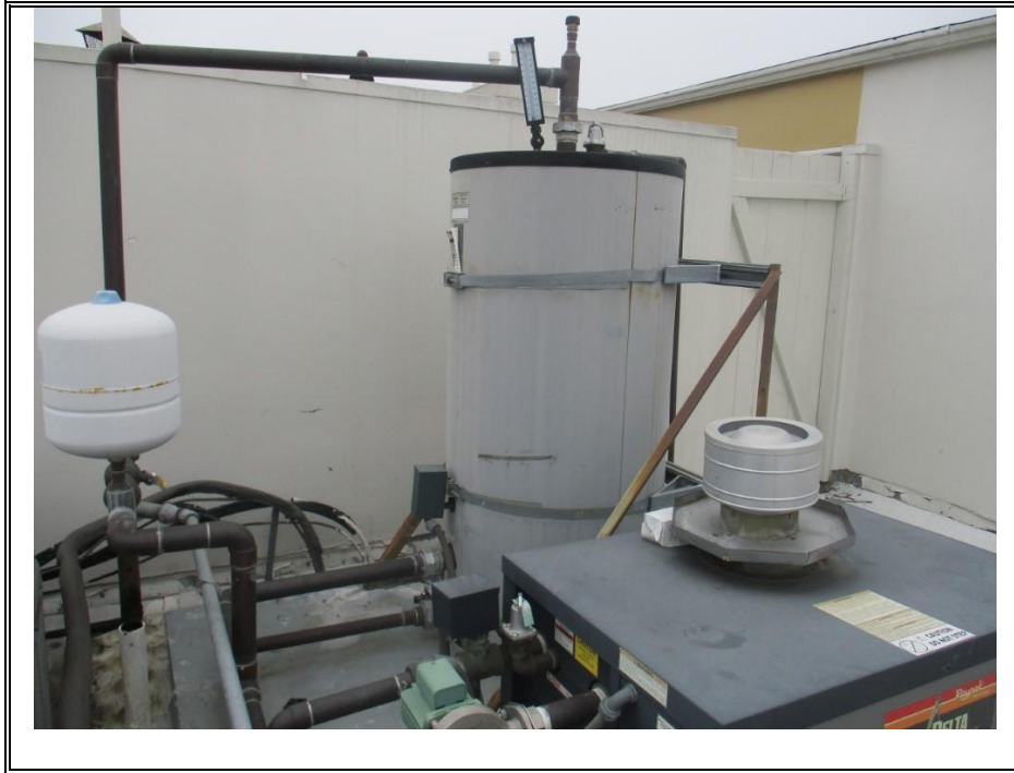
WATER STORAGE TANK (TYPICAL)
