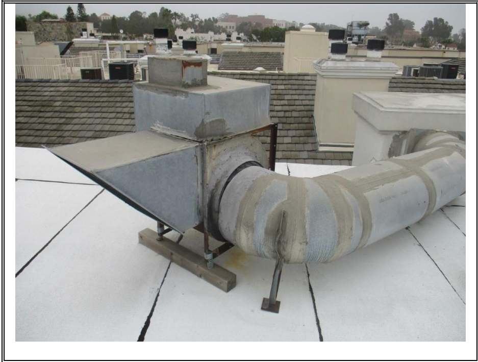
EXHAUST FAN-GARAGE (TYPICAL)
