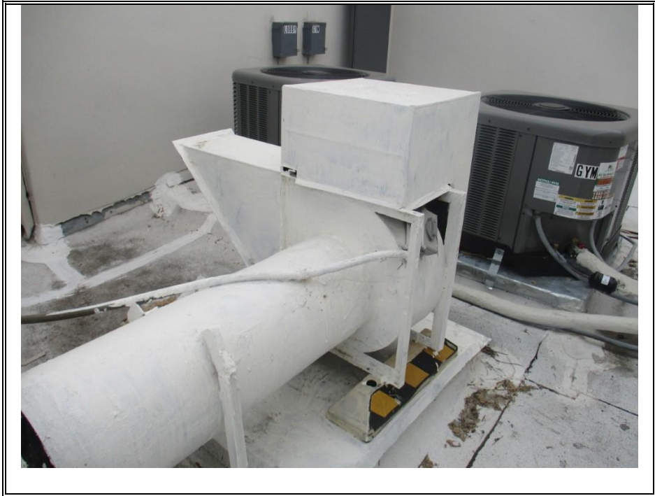
EXHAUST FAN-HALLWAY (TYPICAL)
