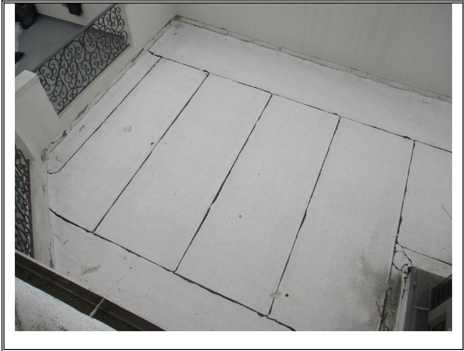
MODIFIED CAP SHEET ROOF (TYPICAL)
