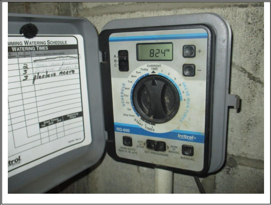
IRRIGATION CONTROLLER (TYPICAL)
