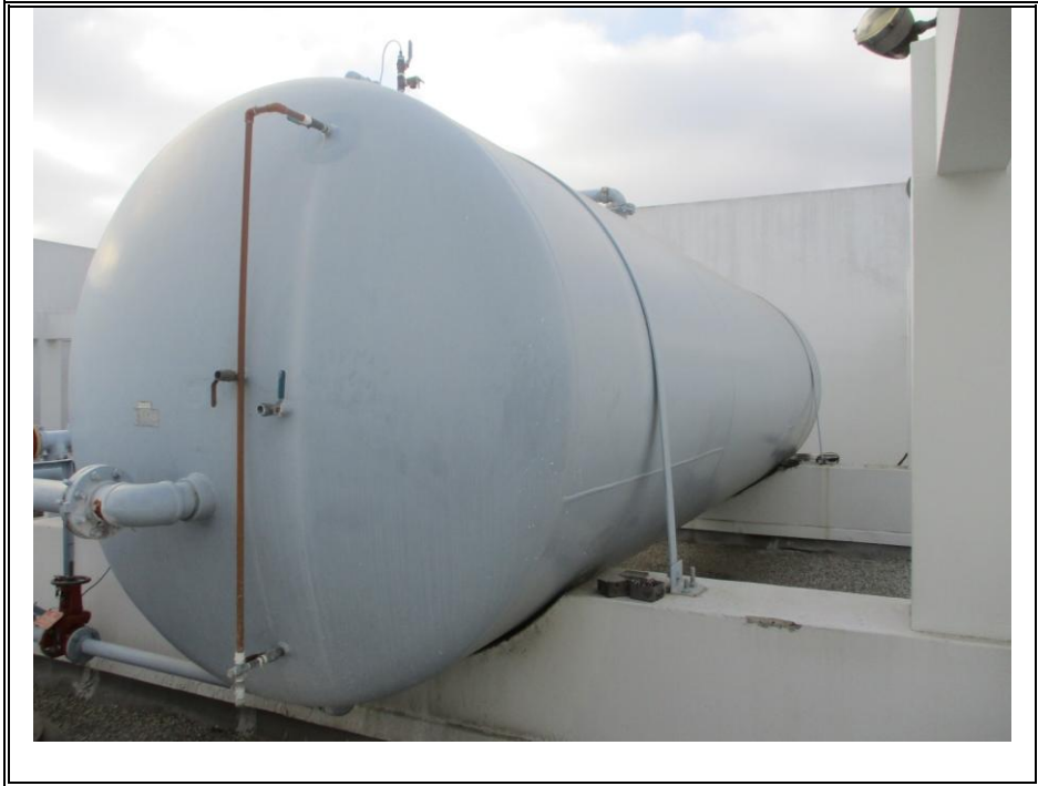
COLD WATER STORAGE TANK-RELINE (TYPICAL)
