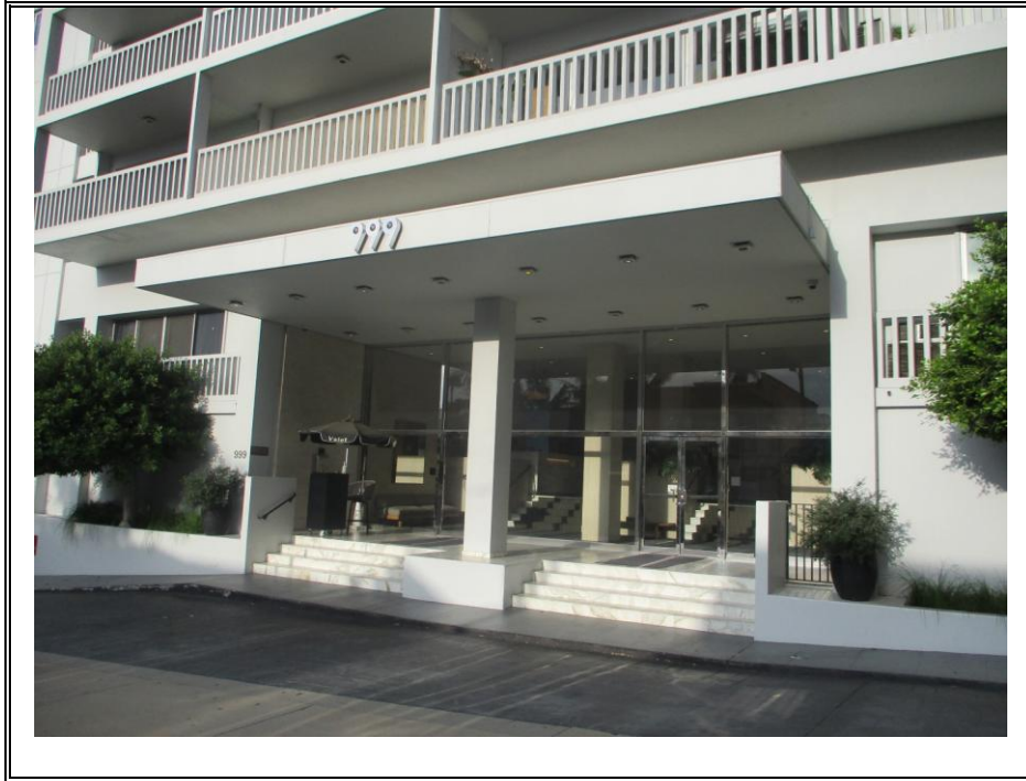
LOBBY ENTRY DOORS (TYPICAL)
