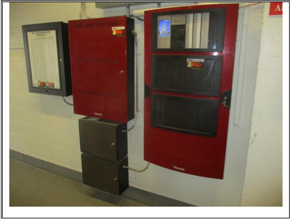
FIRE ALARM SYSTEM (TYPICAL)
