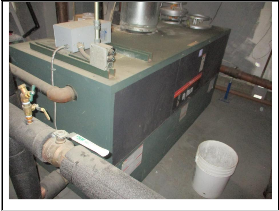
BOILER-OVERHAUL (TYPICAL)
