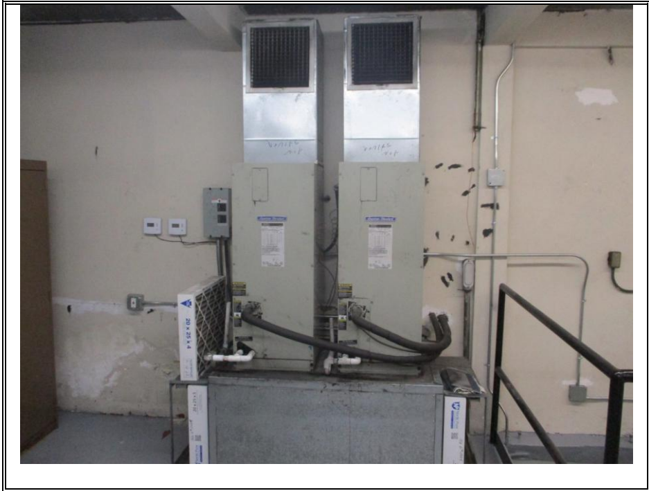
HEAT PUMPS-EVAPORATIVE COILS (TYPICAL)
