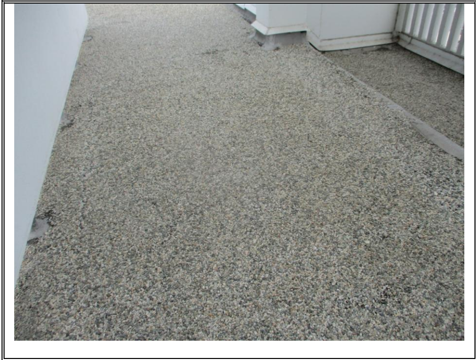
ROOF MAINT/REPAIR/CONSULT (TYPICAL)
