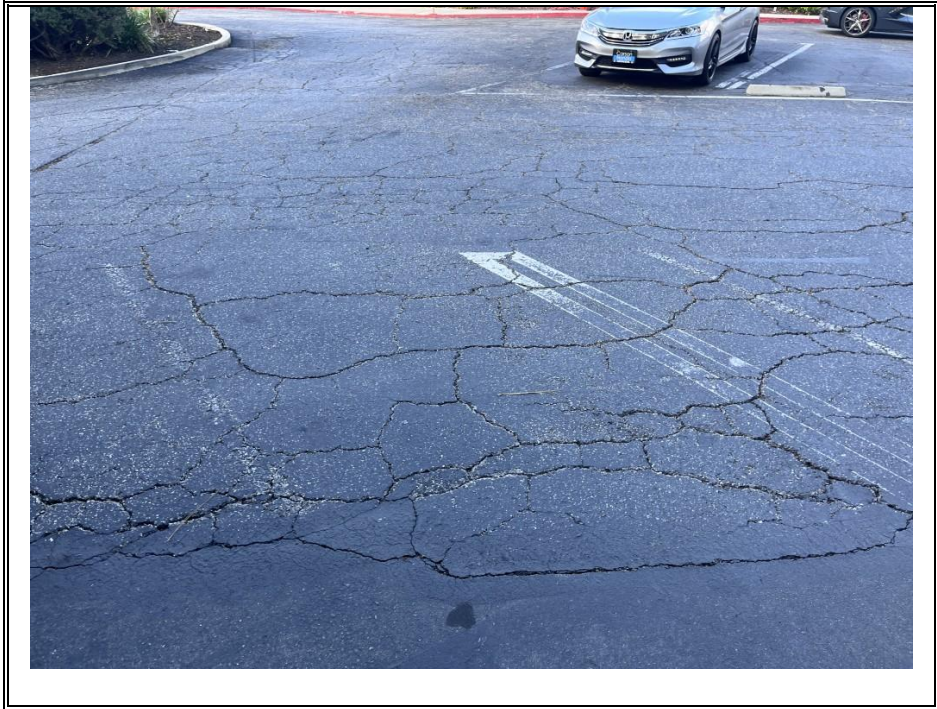
ASPHALT REPLACEMENT (TYPICAL)
