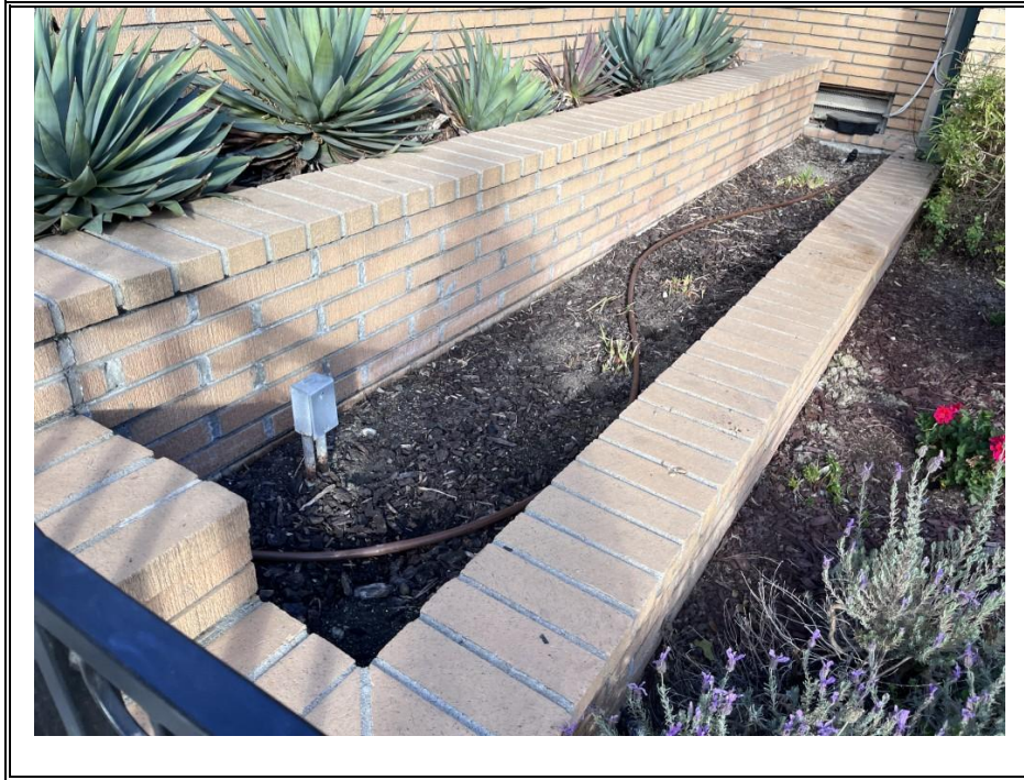
IRRIGATION PIPING (TYPICAL)
