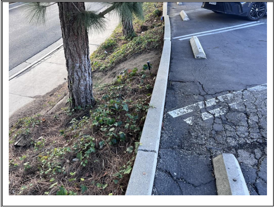
RETAINING WALL-PARKING LOT (TYPICAL)
