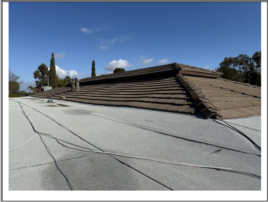
CAP SHEET ROOF (TYPICAL)
