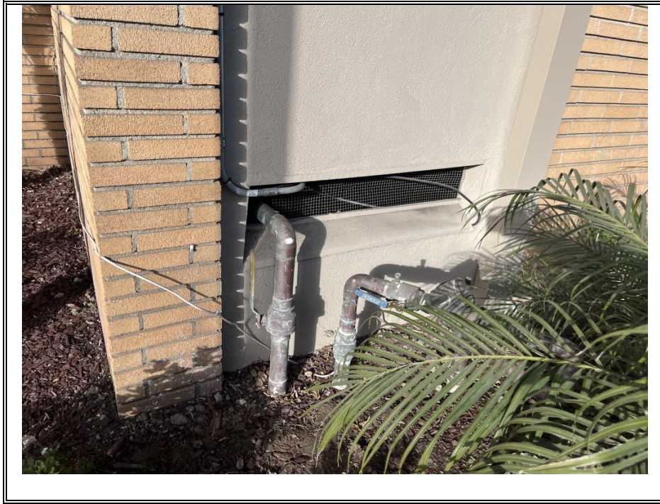
BACKFLOW PREVENTER (TYPICAL)
